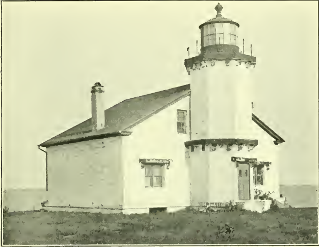
STONINGTON LIGHTHOUSE, BUILT 1842
